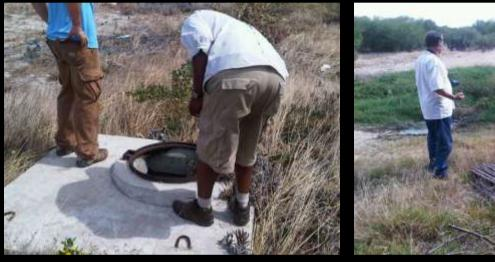
**Figure 22.** One of several uncovered manhole in Fynbos Corridor.
