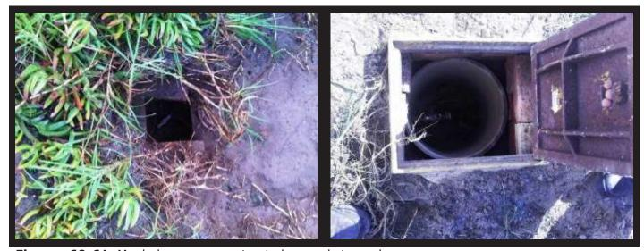
Figures 60-61. Manhole covers constructed around stop valves.
