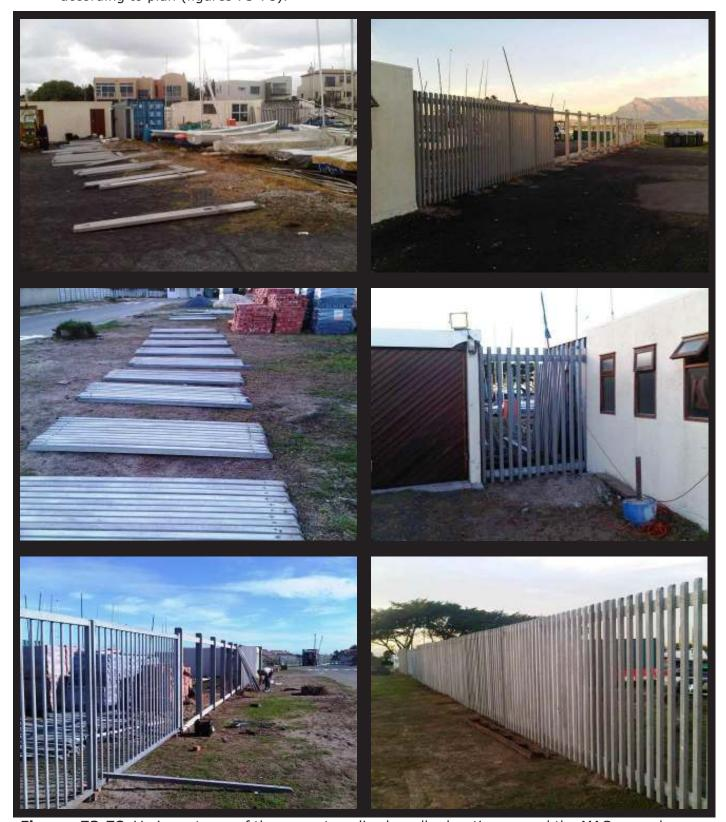
Figures 73-78. Various stages of the concrete palisade wall relocation around the MAC grounds.
