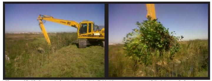
Figures 48-49. Removal of water hyacinth in Table View stormwater outfalls (photos, C. Roux).
