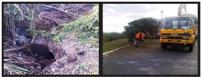
Figure 26. Stormwater outfall pipe opened.
