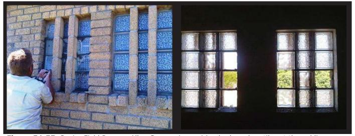
**Figure 54-55.** Senior Field Ranger, Allan Gargan, is repairing broken glass tiles at the public ablution block at Rietvlei.
