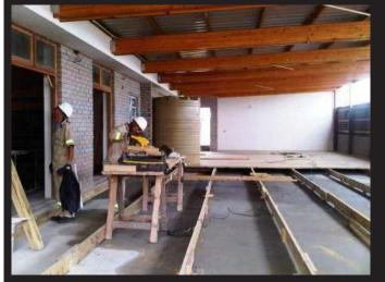
Figure 64. Timber decking in lapa area.
