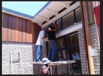
Figure 62. Subcontractor inserting windows.
