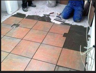
Figure 65. Floor tiling in main office area.
