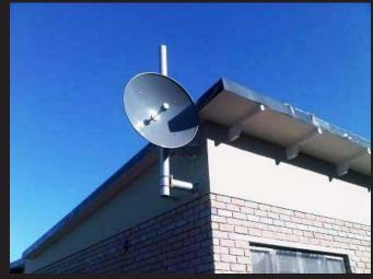
**Figure 63.** Radio receiver dish for City data network.
