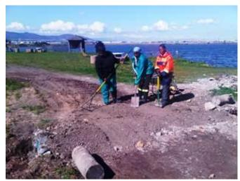
Figure 82. Covering the drainage pipe.
