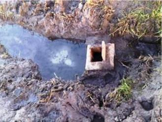
**Figure 85.** Leaking water main at Rietvlei ablution blocked was repaired.
