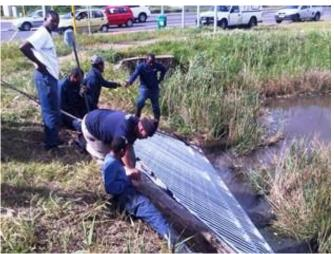
Figure 30. Litter grid inserted at Zoarvlei outlet.
