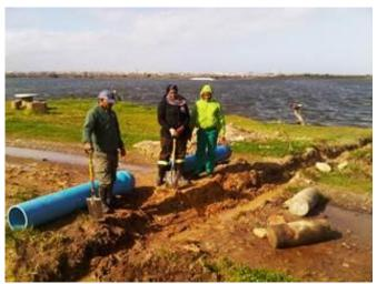
Figure 81. Inserting a drainage pipe.
