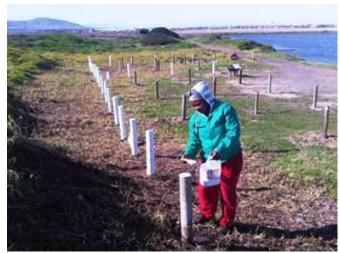
**Figure 89.** Bollard indicating parking areas at fishing sites to prevent damage to shore line.
