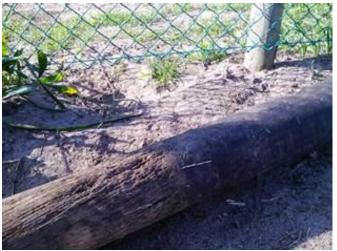
Figure 39. Poles inserted under fence line to stop dogs.
