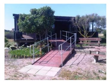
Figure 57. Wheelchair access ramp constructed by the Friends.
