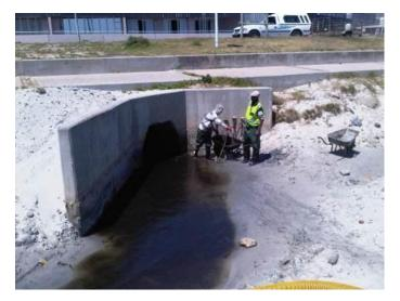
Figure 36. Cleaning of under-road culverts from Zoarvlei.
