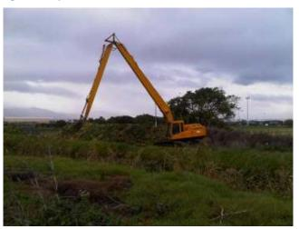
Figure 42. Excavator cleaning Theor Marais Park canal.
