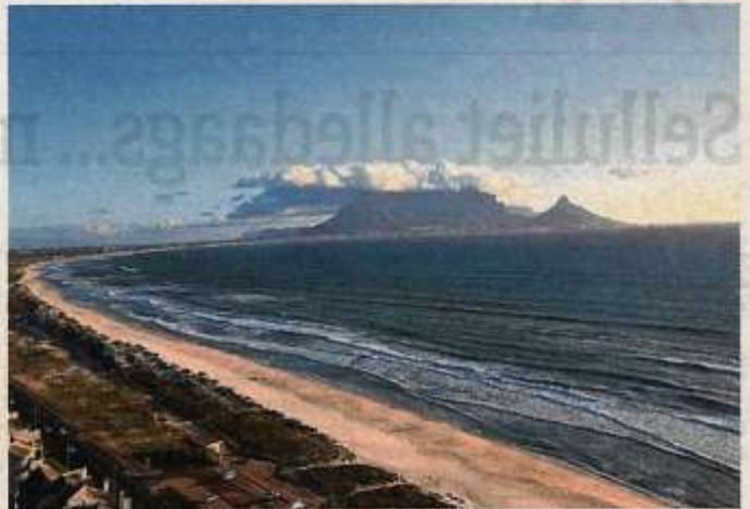
Infrastructure along the Table View coastline is under pressure.
