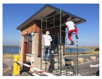
Figure 34. Gate house roof repairs.
