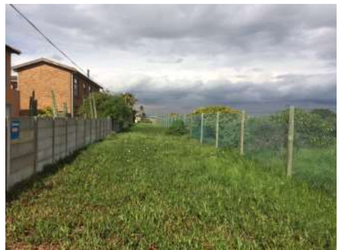
Figure 58. Example of a good firebreak at Sandpiper Crescent.
