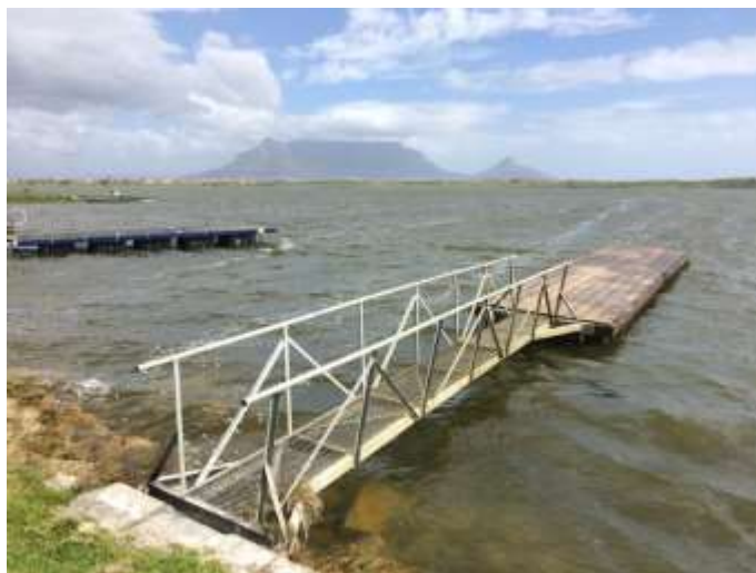
Figure 63. The two jetty panels attached to the catwalk.
