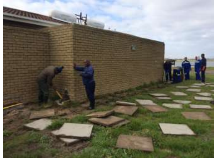
Figure 65. Paving slabs being removed at the ablution block.
