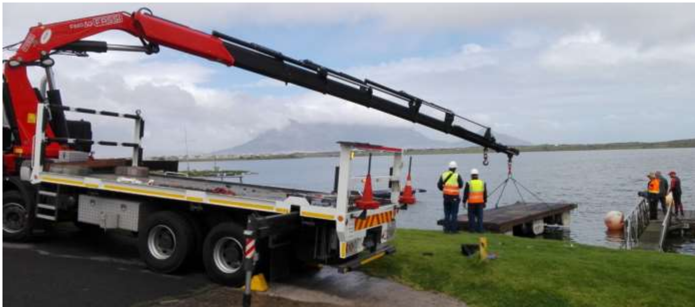
Figure 2. A crane being used to launch the two jetty panels.
