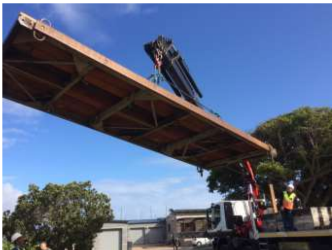
Figure 62. One of the two jetty panels being lifted onto the floats.
