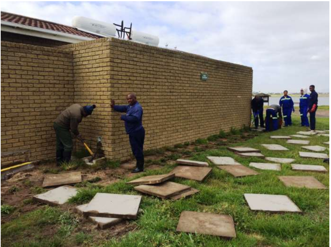
Figure 41. Removal of cement slabs around the Rietvlei public ablution block.
