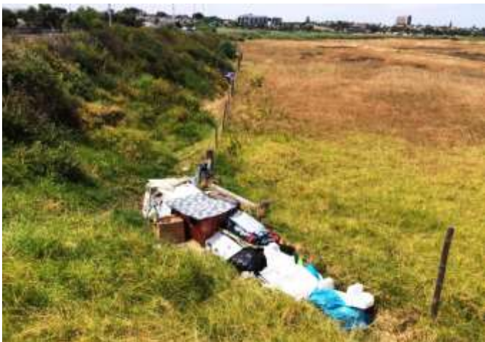
Figure 36. Illegal structures next to the R27 at Milnerton Lagoon.
