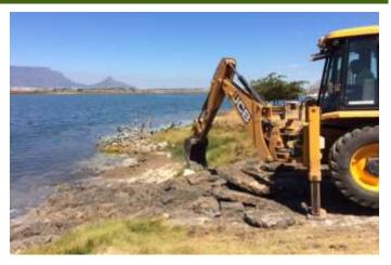
Figure 44. Digger-loader removing the broken slipway near the public ablution block.
