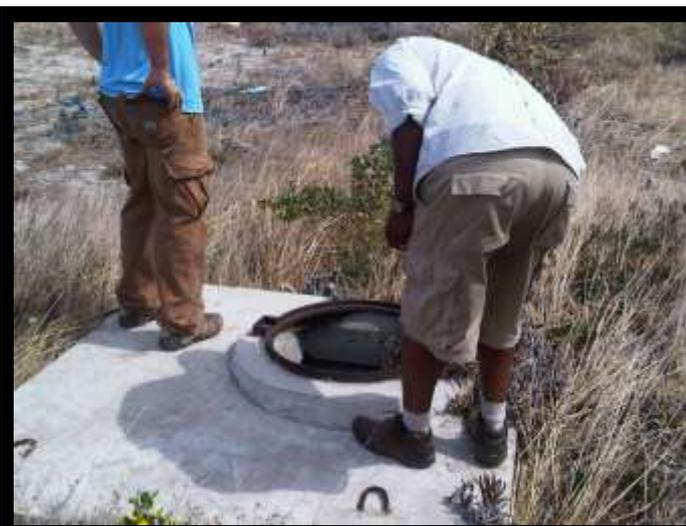
**Figure 22.** One of several uncovered manhole in Fynbos Corridor.
