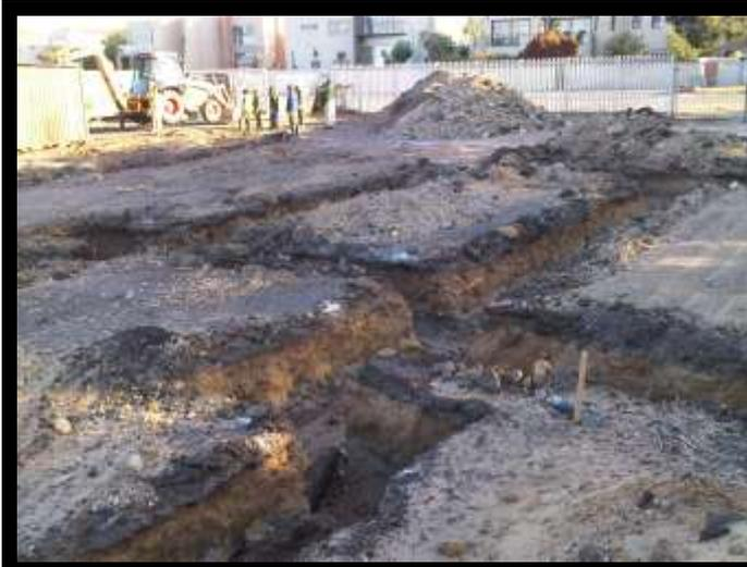
**Figure 43.** Digging of trenches at office construction site.
