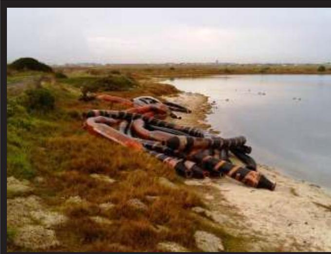
**Figure 54.** Incorrect location of pipe stockpile.
