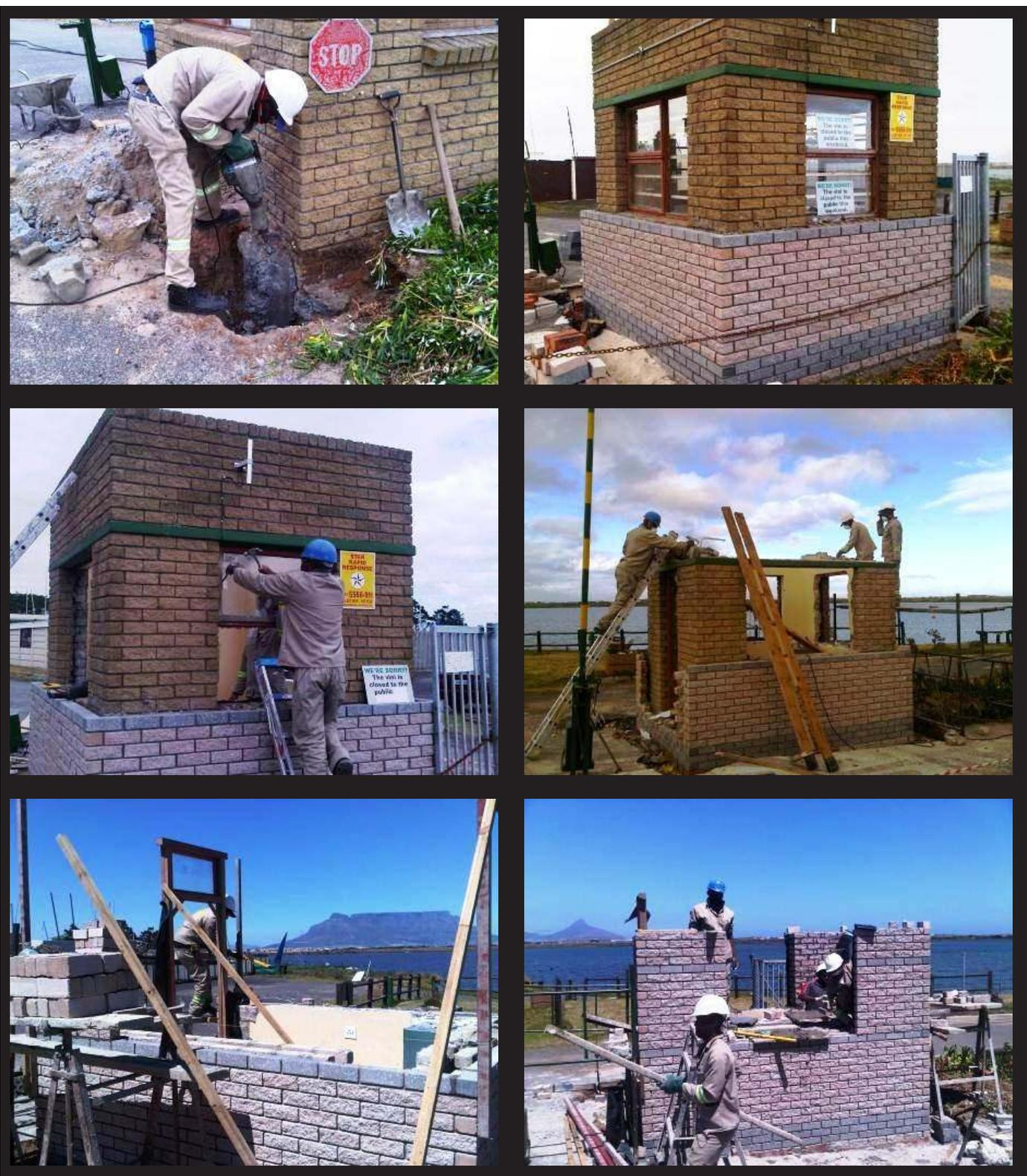
**Figure 68-73.** Various stages of breakdown and reconstruction of the main entrance kiosk (gate house).
