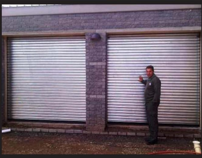
**Figure 77.** Steel roller shutter doors.
