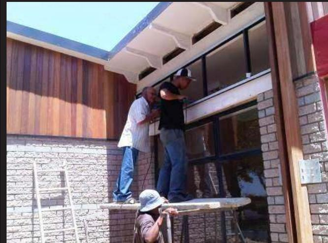
**Figure 62.** Subcontractor inserting windows.
