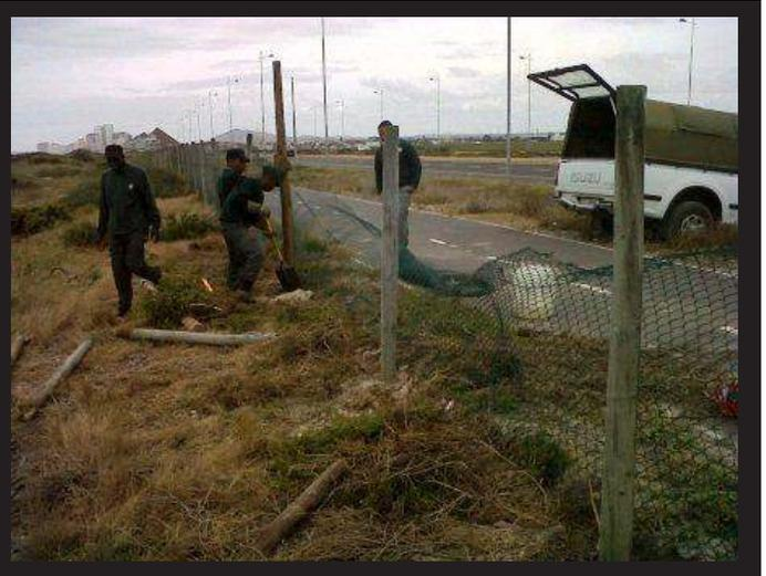
**Figure 53.** Repairs to the Coastal section fence after a traffic accident.
