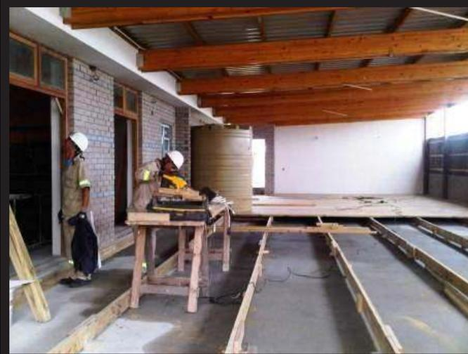
**Figure 64.** Timber decking in lapa area.
