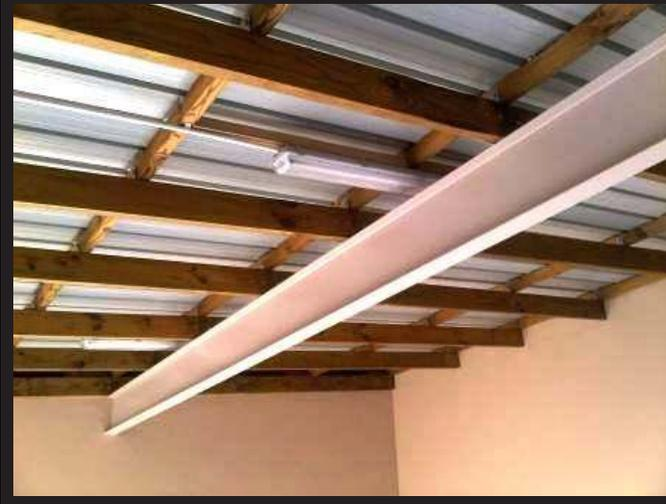
**Figure 74.** Support beam in the triple garage.
