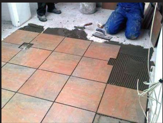
**Figure 65.** Floor tiling in main office area.
