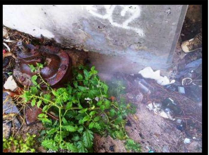
**Figure 26.** A leaking pressure valve detected at Blaauwberg Road bridge, reported and repaired.
