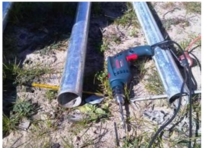
Figure 95. Drilling of holes and inserting of steel pegs in the base of the pole to prevent removal from concrete.
