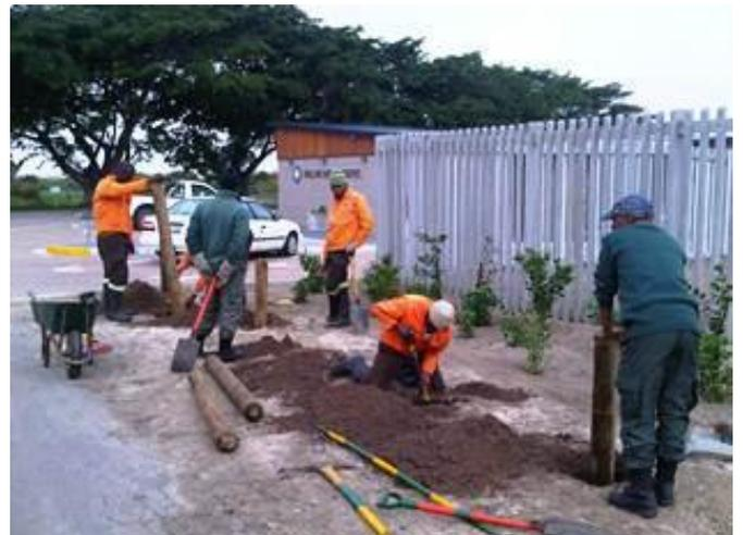
**Figure 91.** Planting of bollards around the office.
