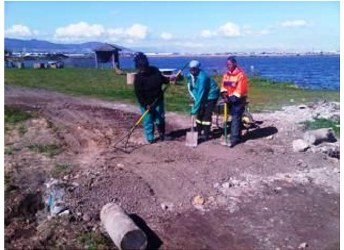
**Figure 82.** Covering the drainage pipe.
