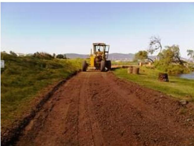
**Figure 84.** Tourist road at Rietvlei being scraped by the Roads Department depot machinery.
