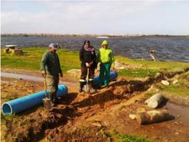
**Figure 81.** Inserting a drainage pipe.
