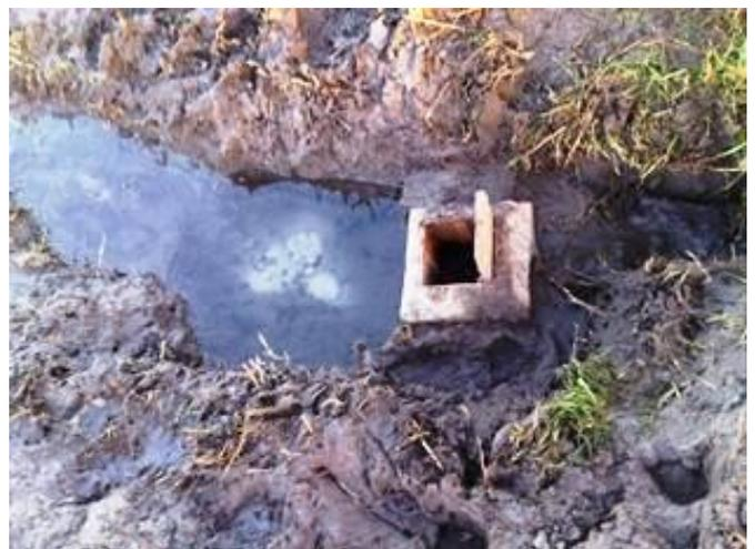
**Figure 85.** Leaking water main at Rietvlei abluition blocked was repaired.
