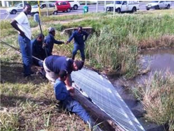
**Figure 30.** Litter grid inserted at Zoarvlei outlet.
