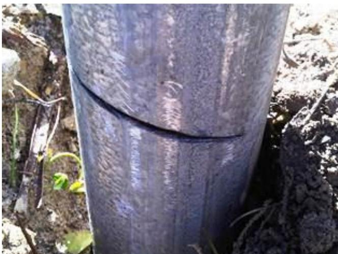
**Figure 55.** Vandals not able to cut through sign post.
