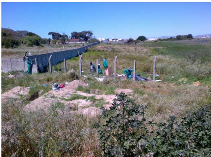
Figure 49. The vibracrete wall being removed (photo by C. Roux).
