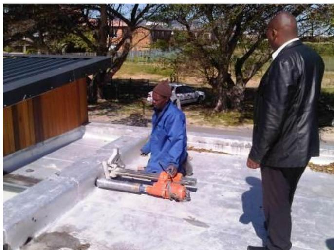
Figure 81. Contractors repairing waterproofing at Rietvlei office.
