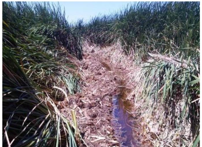
Figure 16. Cutting of drainage channels through reeds.
