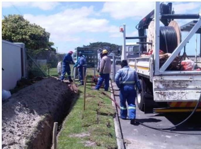
Figure 79. Eskom cabling being laid.
