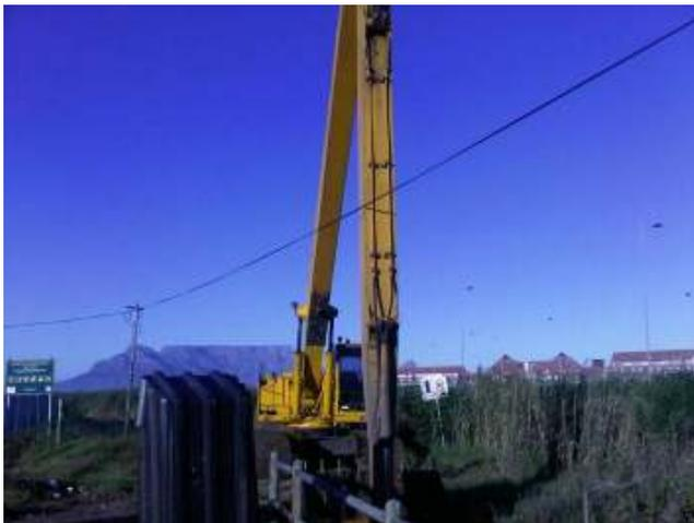
Figure 41. Excavator cleaning Bayside Canal.
