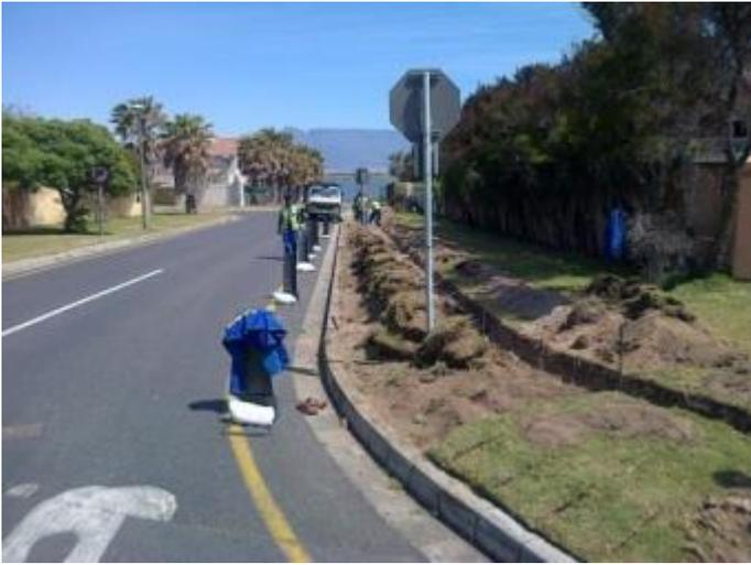
Figure 46. Construction of a section of the pavement sidewalk.
