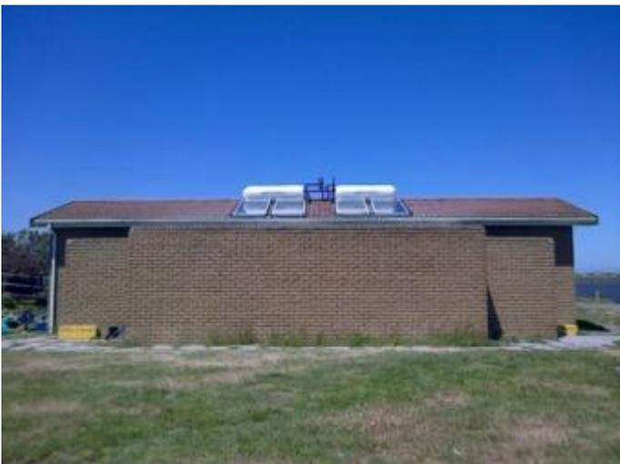
Figure 50. Solar geysers installed at ablution block.
