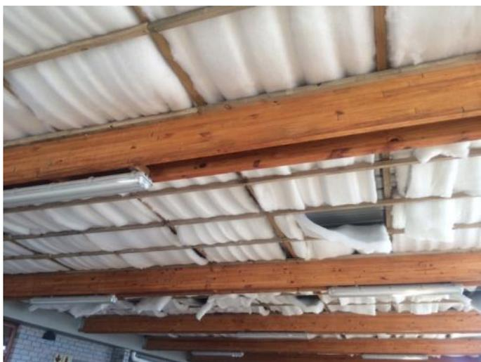
Figure 47. Ceiling insulation work in progress.
