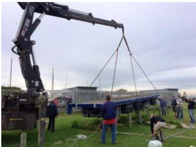
Figure 36. The Milnerton Aquatic Club's new jetty being launched with the help of a crane truck hired by the Club.
