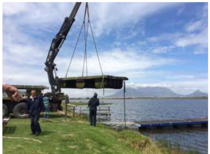
Figure 37. One of the two portions of the Nature Reserve's old Council jetty being taken out of the water for repairs.
